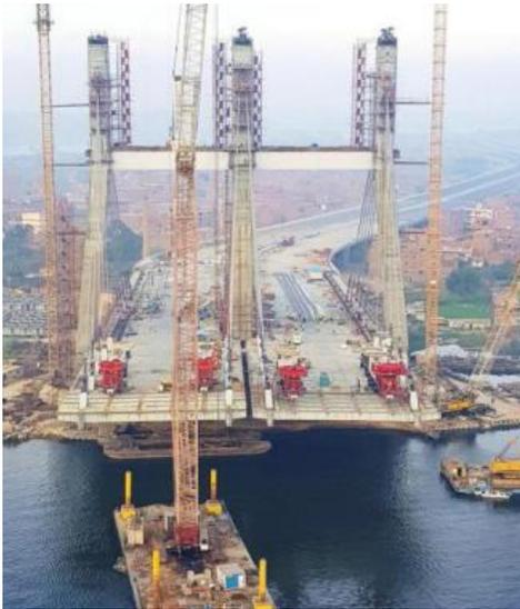
Several custom-made crane barges were built just for the Rod el Farag Axis Bridge construction project. Six 92 m tall towers support 160 cables. The concrete towers were protected with Xypex Concentrate.
