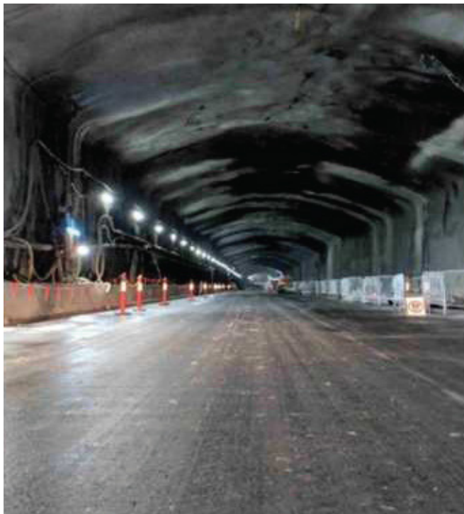
Westconnex Tunnel Construction.
