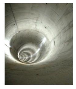
The Thames Tideway Tunnel is London's new "super sewer" running from Acton to Abbey Mills. It is being built to prevent millions of tonnes of pollution reaching the River Thames. Xypex was used within the west section of the tunnel and is the sole waterproofer for the Hammersmith Connection Tunnel.
