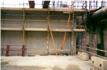
A combination of Xypex products was used to repair and waterproof the main service tunnel connecting Terminal 5 at Heathrow Airport with other terminals. Repairs with Xypex Concentrate and Patch'n Plug were so successful that Xypex Admix was specified on all remaining cast-in-place concrete. Over 5 tonnes of Xypex Admix C-1000 NF has been used to date on this project.
