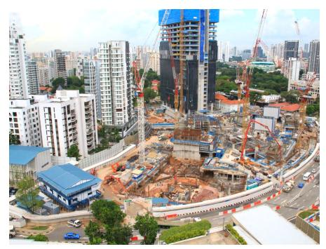
Both Xypex Admix C-1000 NF and Xypex Concentrate were used in the 19,000 m $^2$  4th level basement slab and skin walls as well the underpass link base slab, walls, and roof. A total of 58,500 m $^3$  of concrete were treated in all. Construction joints were treated with Xypex Concentrate.
