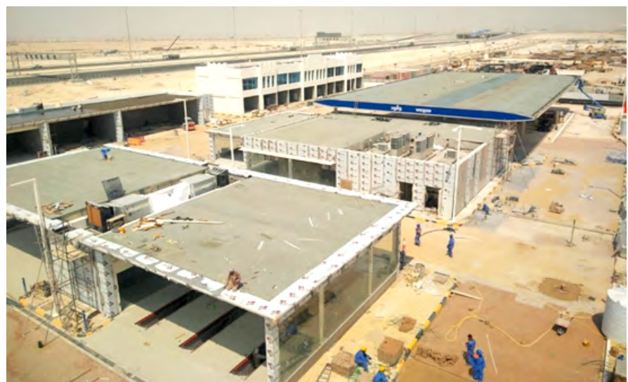
Slab on grade casting
