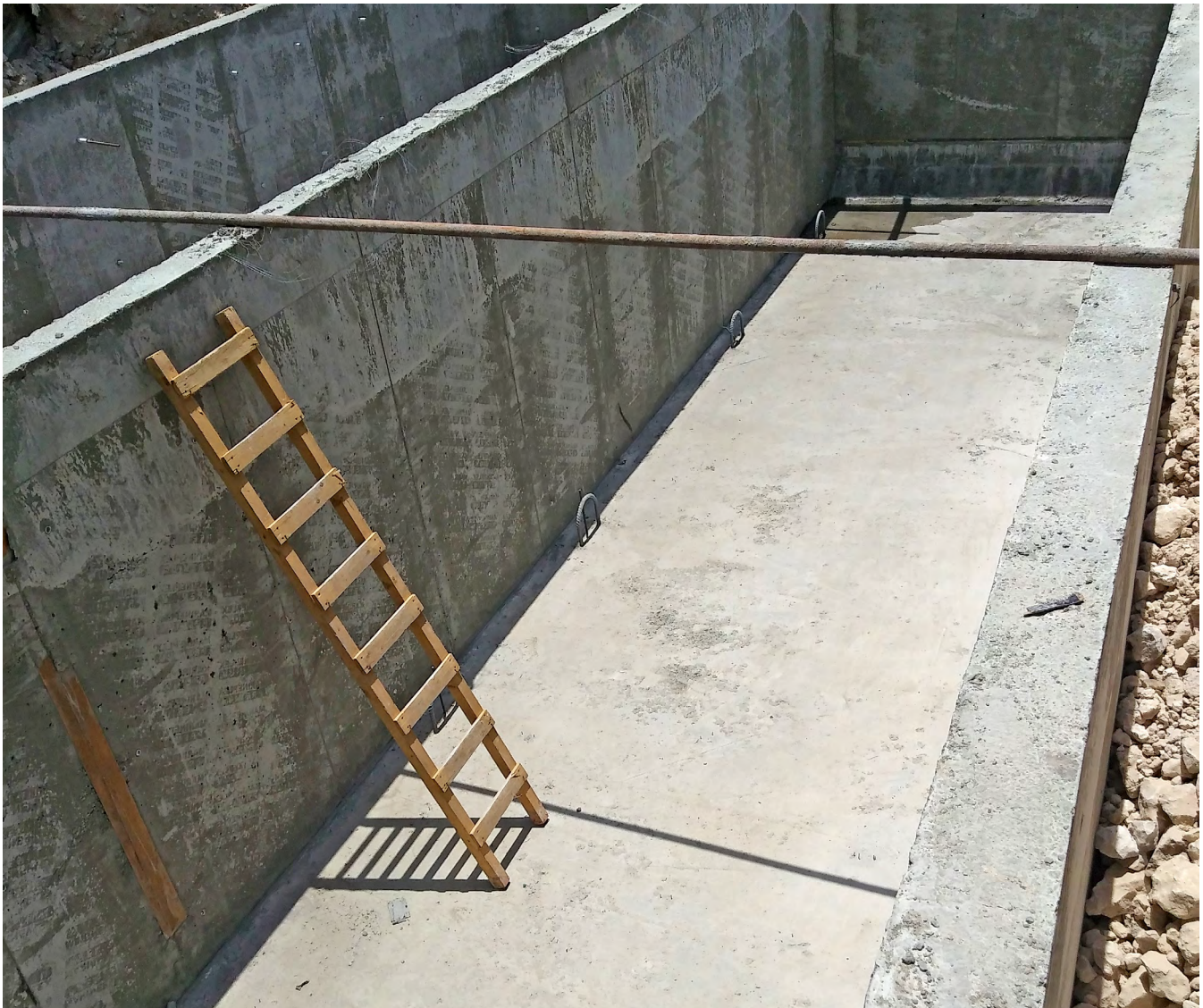
Fuel tanks cast with Xypex Admix C-1000 NF
