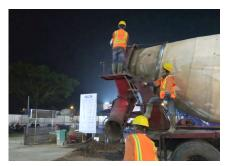
Mixing Xypex Admix into the concrete truck
