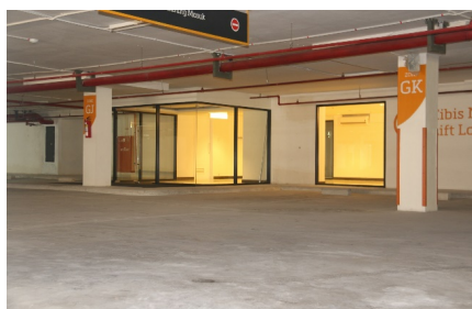
Top: before repairs Bottom: after Xypex application
