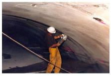
Commencing in September of 1991, repair systems using Xypex Concentrate and Patch'n Plug were used as part of an ongoing program of repair and maintenance of the North and South land driven tunnels and transition tunnels of this renown structure. Xypex products were selected ahead of some 52 others to repair the extensive cracking that has occurred.
