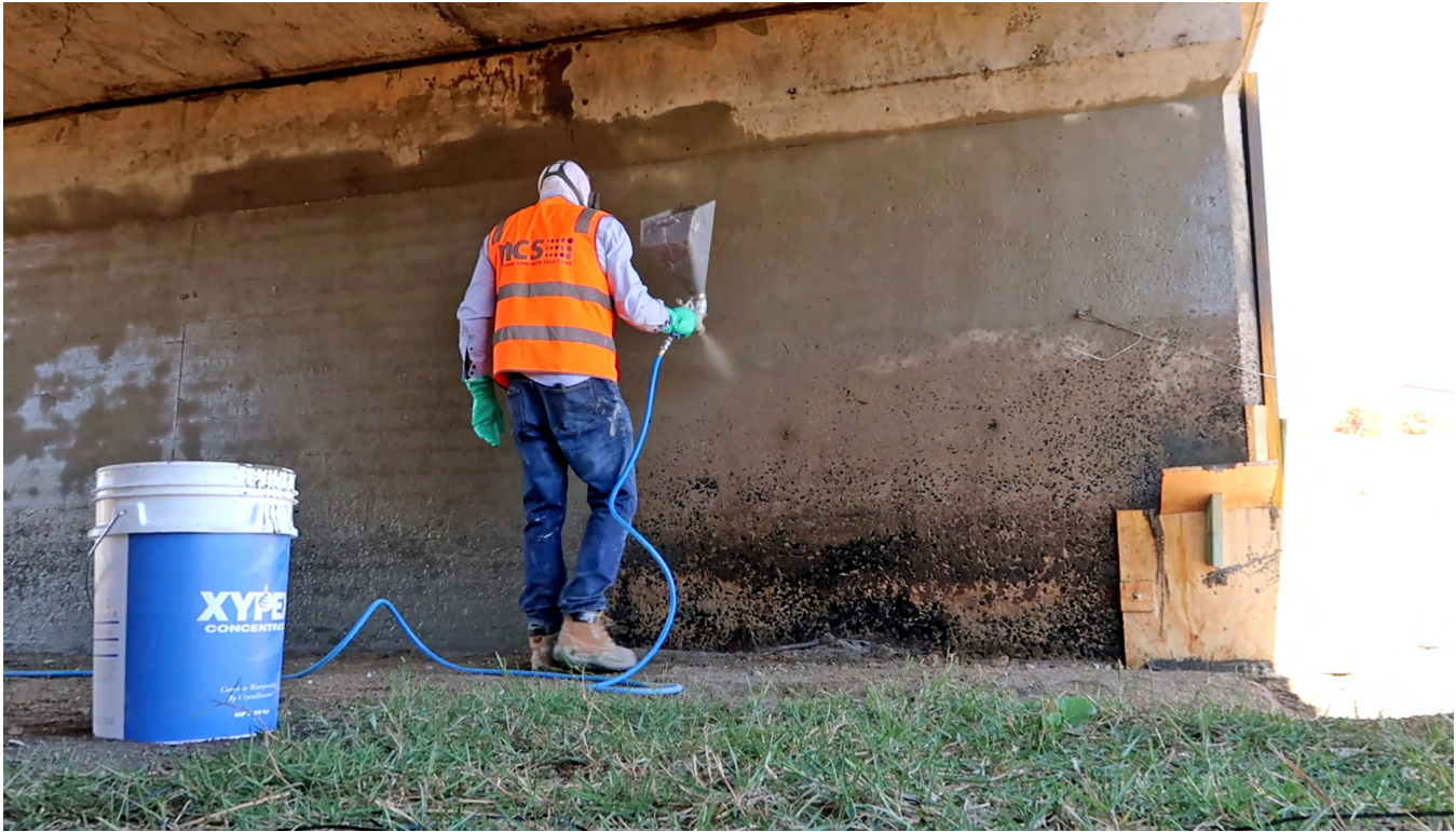
Spray Application of Xypex Concentrate
