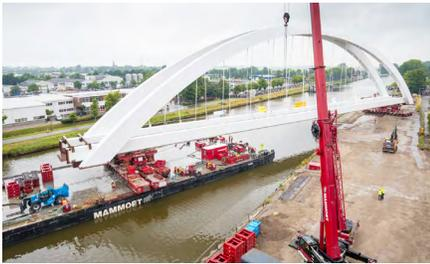
Fig 2 -- An assortment of heavy lift technology is employed by the Mammoet company in order to move one end of the 1,700-ton steel bridge across the canal and into its final position.
