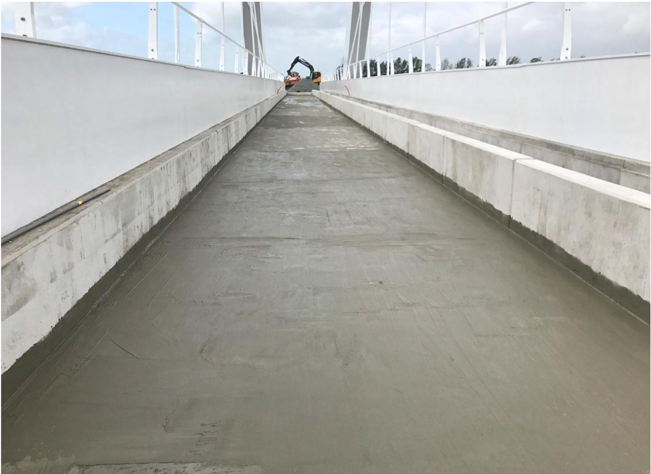
*Fig 7 -- Xypex Concentrate has been applied to the concrete deck of the new Zuidhorn railway bridge, creating an integral bond and protecting the concrete from moisture and harsh chemicals.*
