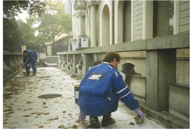
The contracting company responsible for the work was ABV s.r.o. Praha 9. Xypex Concentrate, Xypex Modified, and Xypex Patch'n Plug were selected to waterproof the ancient masonry. These Xypex products provided the project with a permanent waterproofing solution, playing a crucial role in enhancing the waterproofing capabilities of the bridge and contributing to its preservation and longevity amidst its high-profile location.
