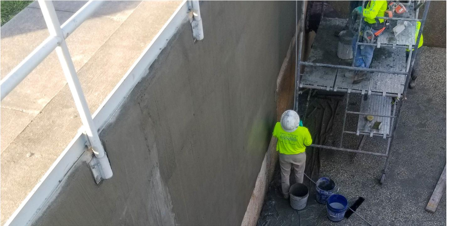
View of the sludge tank undergoing repair with Xypex Megamix II with BioSan.
