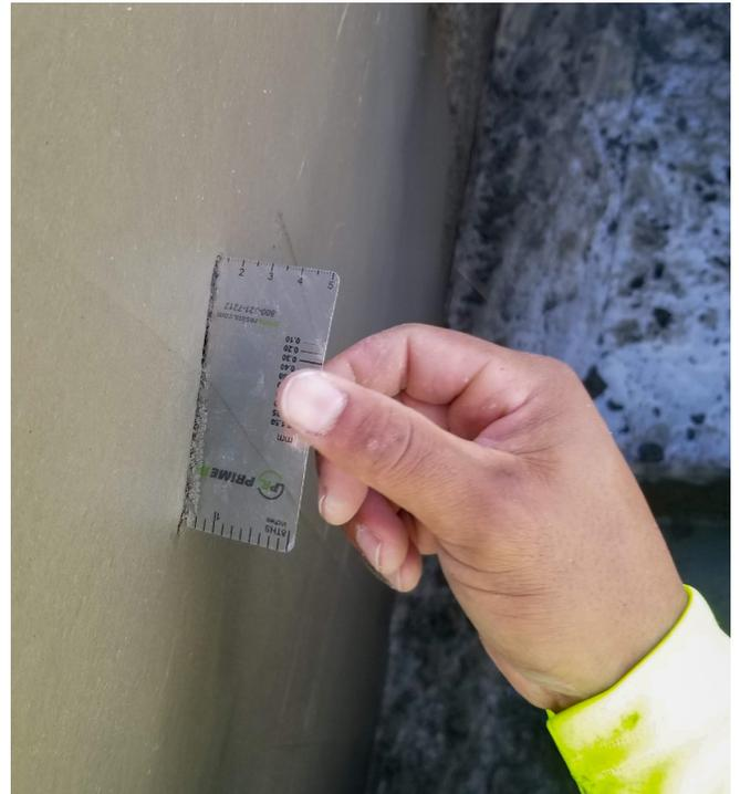
To ensure the correct application and durability of the product in the elements, the thickness of the coating is continuously verified, ensuring its performance in the future.
