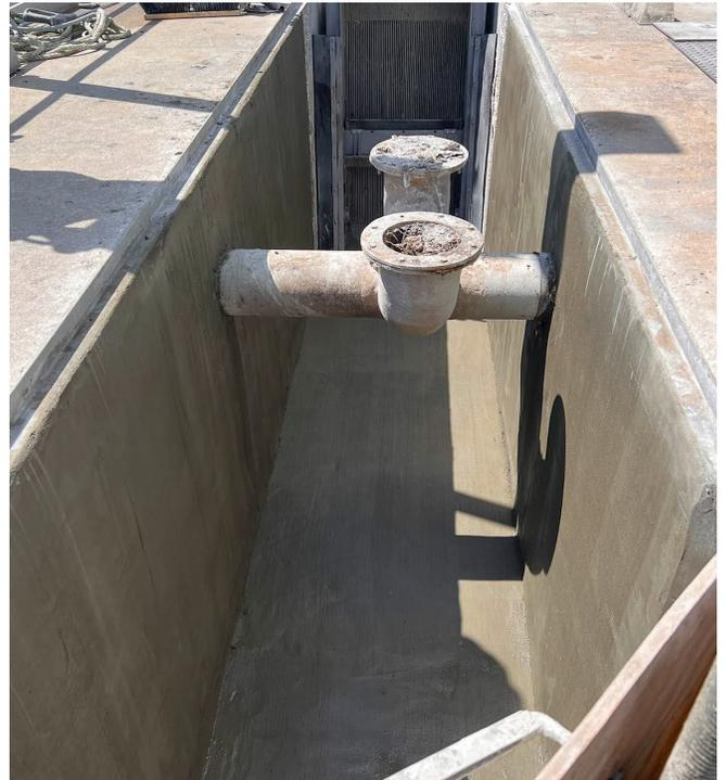
The maintenance pit was repaired with Megamix II with Bio San, thus extending the service life of the concrete structure.
