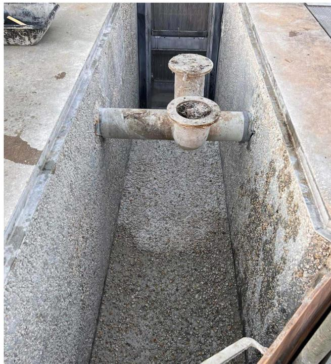
The concrete shows severe damage in the maintenance pits caused by Microbial-Induced Corrosion (MIC), reducing the service life of the structure.
