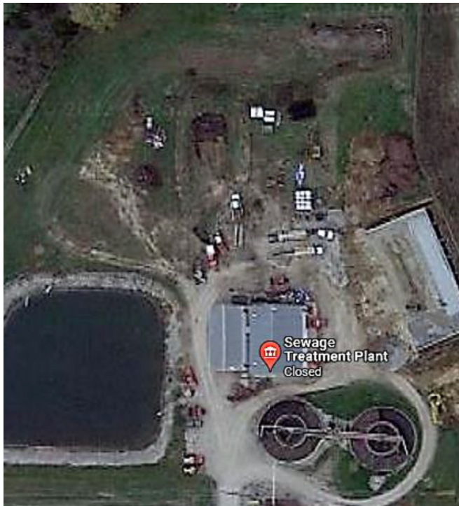
Aerial Google street view shot of the sewage treatment plant.
