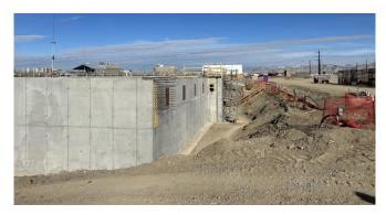
As part of the expansion, Xypex Admix C-500 was incorporated at the time of batching into the concrete used for the facility's new water-holding structures. By integrating Xypex directly into the mix, the need for traditional surface-applied waterproofing methods was eliminated, resulting in significant cost savings and long-term durability.
