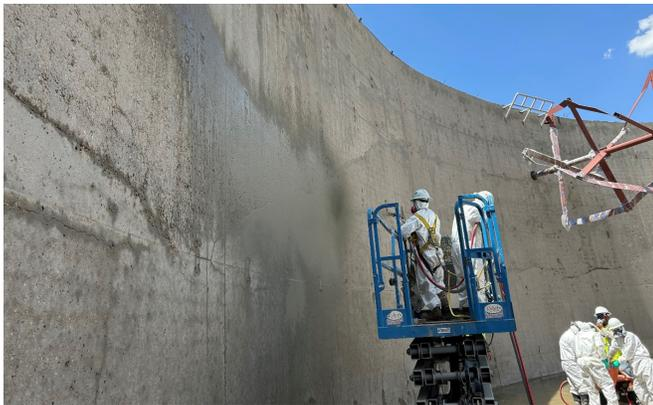
Sunland Construction, the general contractor, self-performed the application across six tanks using Xypex Concentrate (primary waterproofing), Xypex Modified (enhanced protection in high-stress zones), and Xypex Patch'n Plug (for crack repair prior to treatment).
