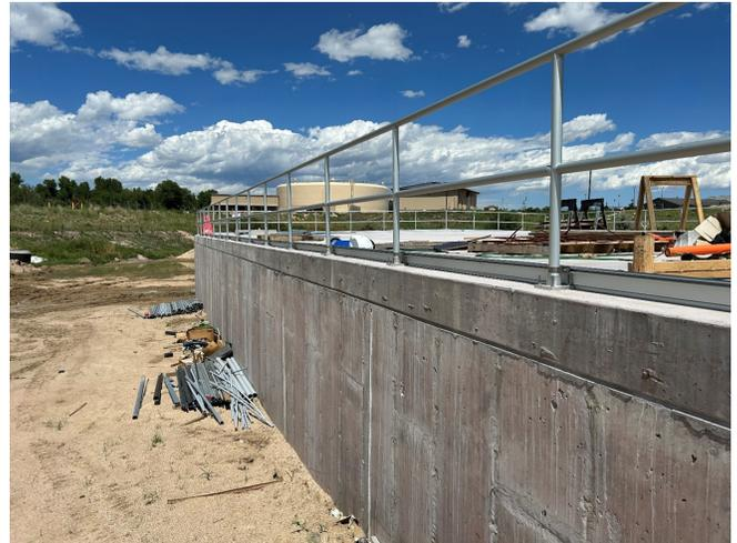
To address the harsh conditions within the lift station, Xypex Bio-San was incorporated into the concrete mix, providing integral protection against microbial-induced corrosion (MIC) caused by high levels of hydrogen sulfide (H<sub>2</sub>S). Its advanced crystalline technology enables self-healing of micro-cracks and resistance to hydrostatic pressure, ensuring long-term impermeability and structural integrity.
