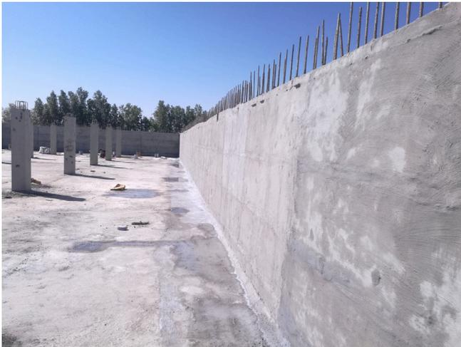
Xypex Concentrate was applied to the interior surface of the treatment tanks spanning 2,289 m<sup>2</sup>. Xypex Concentrate penetrates into the concrete where it chemically reacts, forming an insoluble crystalline structure that seals micro-cracks and capillaries, preventing water ingress. The Xypex crystalline also increases the concrete's chemical resistance by significantly reducing the ingress of deterioration causing substances like chlorides and sulphates.
