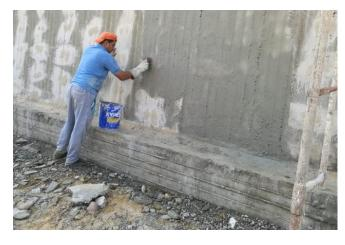
Its chemical resistance safeguards structural integrity against harsh conditions, and its flexibility in application—on both positive and negative sides of concrete, without needing a dry surface—facilitates efficient installation. Environmentally safe, non-toxic, and VOC-free, Xypex Concentrate provides a permanent, maintenance–free solution that is cost-effective and extends the concrete's service life, aligning with the project's sustainability and durability objectives.
