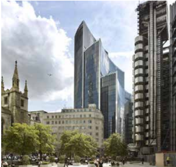
Willis Building, London, England
