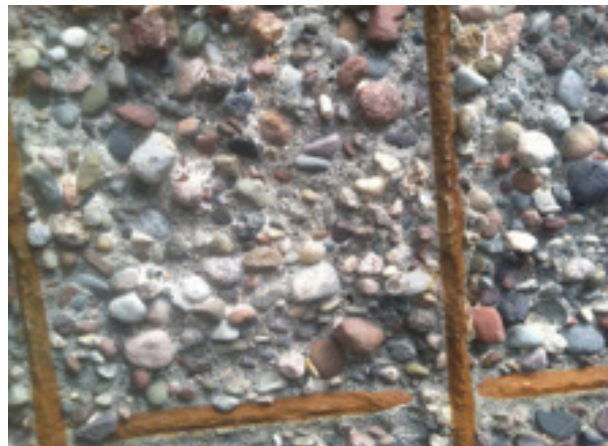
MIC deterioration at a wastewater treatment plant intake structure with a loss of approximately 2" of concrete.
