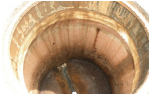
Terrebonne Parish manholes with crystalline admix show little deterioration after 10 years of service.
