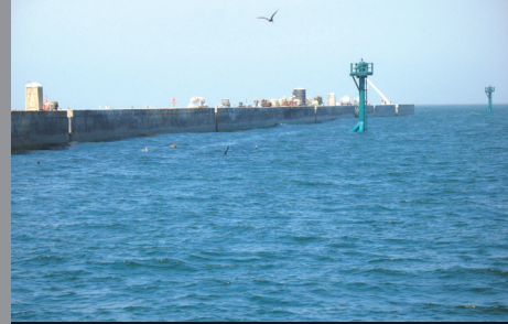
Sempra Energy Breakwater, Mexico
