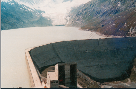
Grimsel Area Dam System, Switzerland
