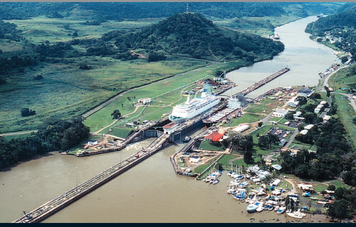
Panama Canal: Chamber Wall of Gatun Locks, Panama
