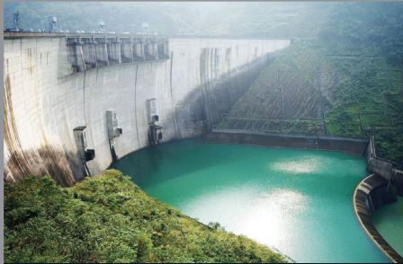
Taipei Feitsui Reservoir, Taiwan
