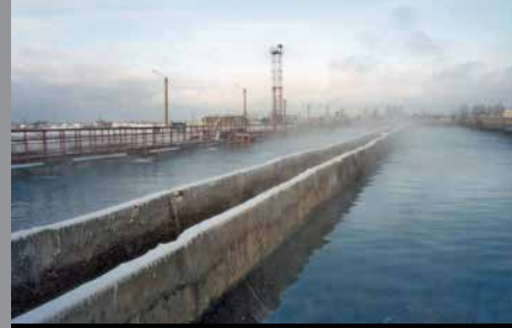
Novgorod WWTP, Russia
