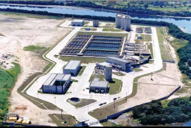
Allegria WWTP, Brazil
