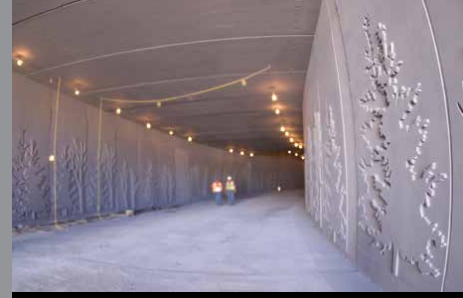
Bremerton Tunnel, USA
