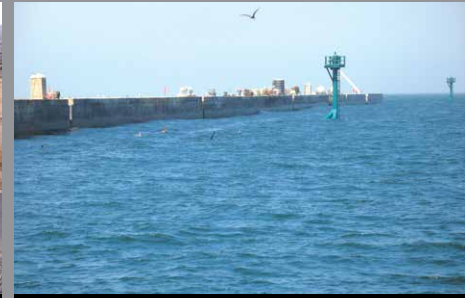
Sempra Energy Breakwater, Mexico
