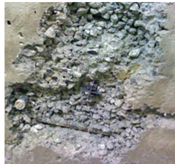
Construction defects (rock pockets, honeycombs & untreated tie holes)
