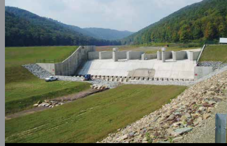
Lyman Run Dam, USA
